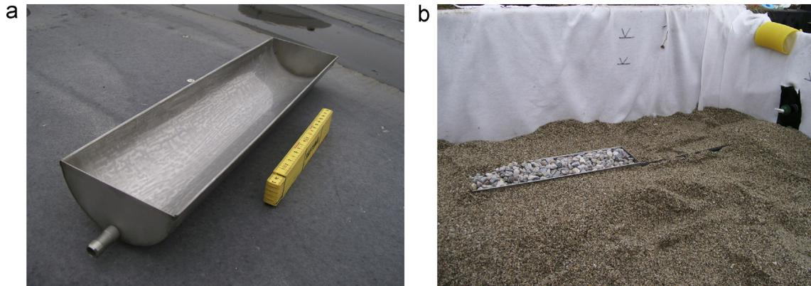
Fig. 18. Internal interception pans in the unsaturated vertical flow beds (VS1, VS1p, VS2, VS2p, VG, and VGp): (a) before installation and (b) during installation.
