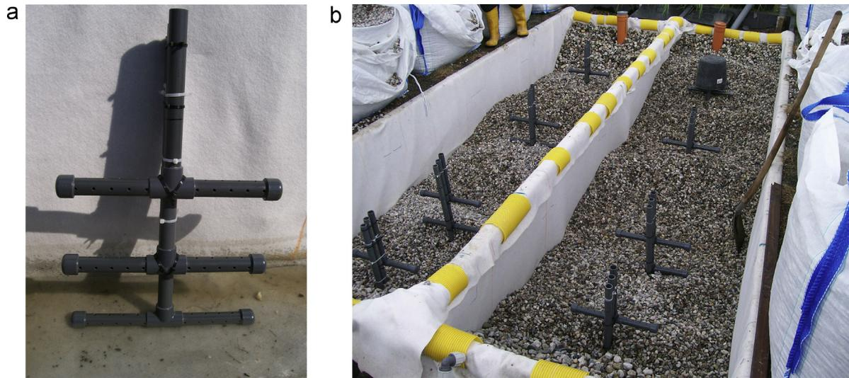
Fig. 12. Internal sampling tees for saturated beds: (a) before and (b) during installation.
