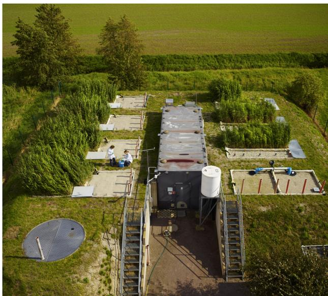
**Fig. 1.** The Langenreichenbach ecotechnology research facility in Germany. The system abbreviations, starting from the bottom left hand corner and going clockwise are: VS2, VS1, VG, VA, HA, H25, H50, and R. All systems with the exception of the last were installed in pairs (one planted with *P. australis*, the other left unplanted).
