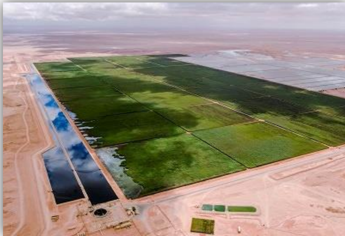
Plate 1: System in Oman treating >100,000 ML/d of oilfield wastewater, with 350 ha Surface Flow Wetlands and 450 ha of ponds. Dr Tom has been involved with the design, construction, vegetation management and operation of the facility since 2011.
