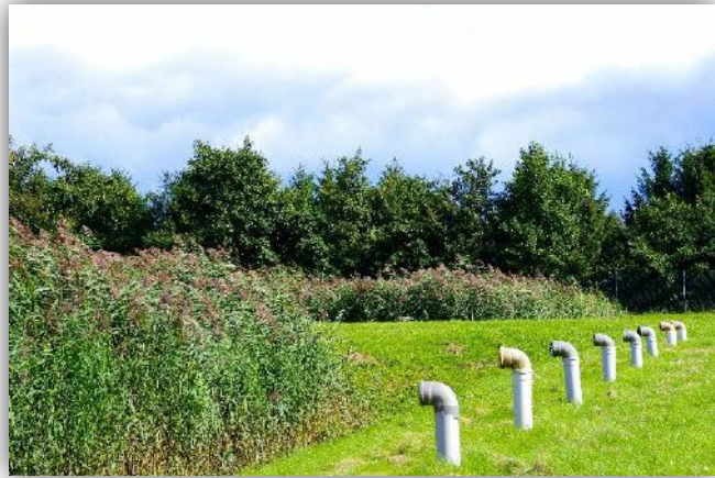
Plate 2: A Sludge Treatment Wetland system in Denmark operating for 20 years, converting waste activated sludge into stabilised biosolids.
